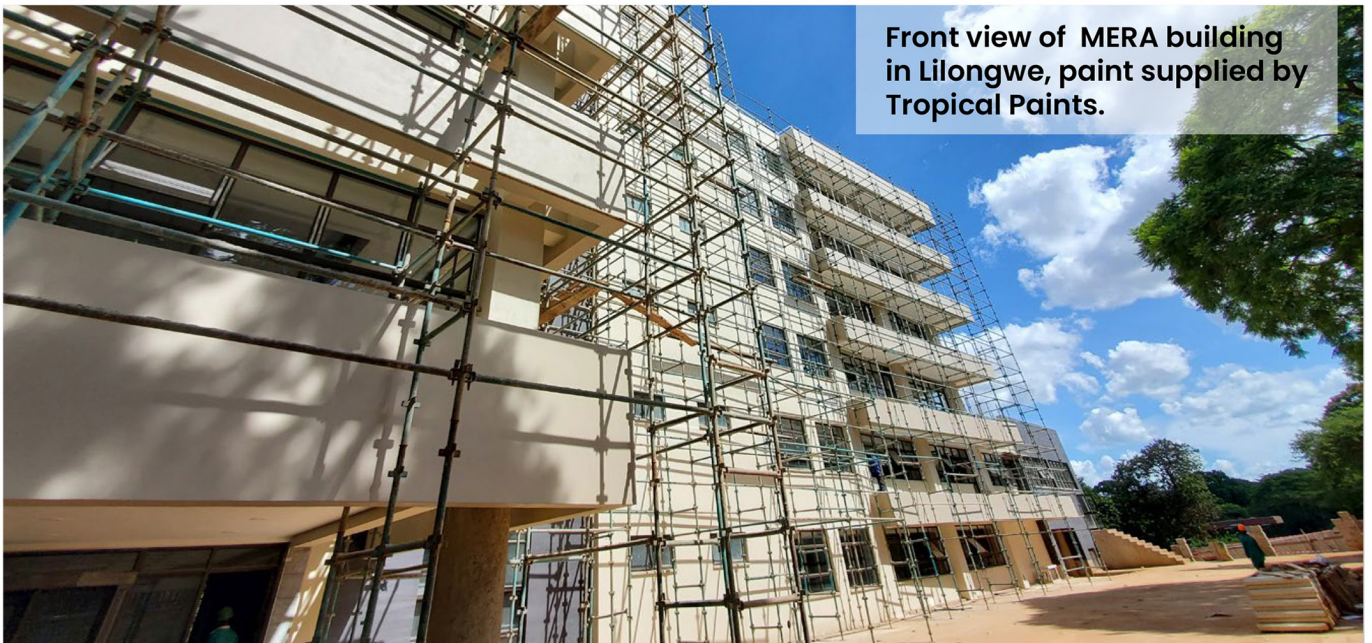
MERA building in Lilongwe, Paint supplied by Tropical Paints.
